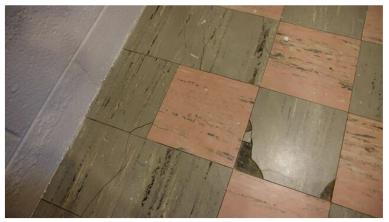
Figure 67: Asbestos containing products
