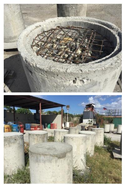
Figure 74: Diagrams and photos showing outer liner with reinforcing metal and final concrete finish of the culvert encapsulation
